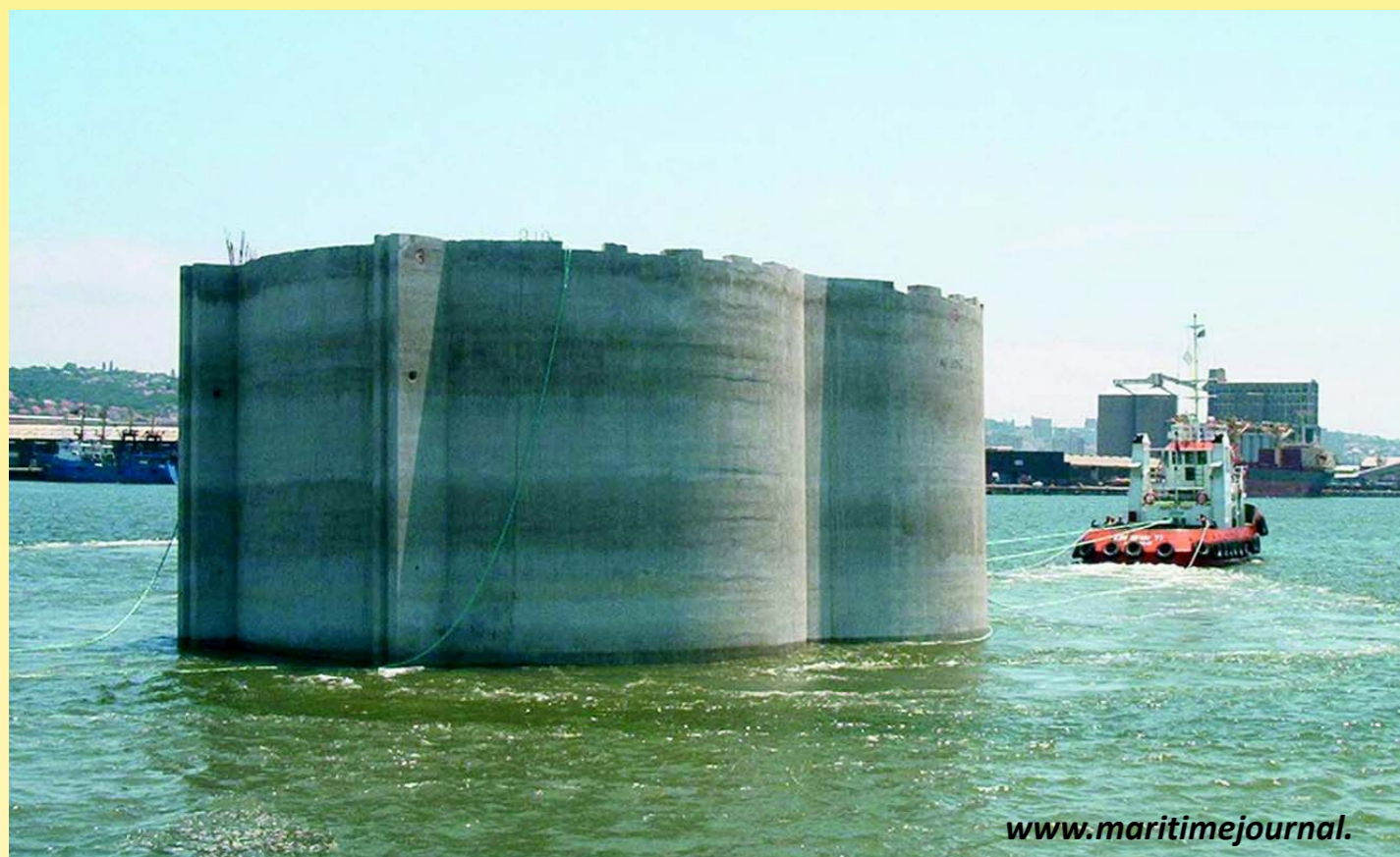
Physical flexibility: Caisson being towed
